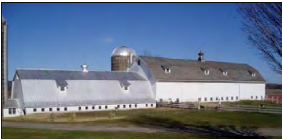
The barn houses the milking parlor, milk house, cheese processing rooms, coolers and aging caves.
